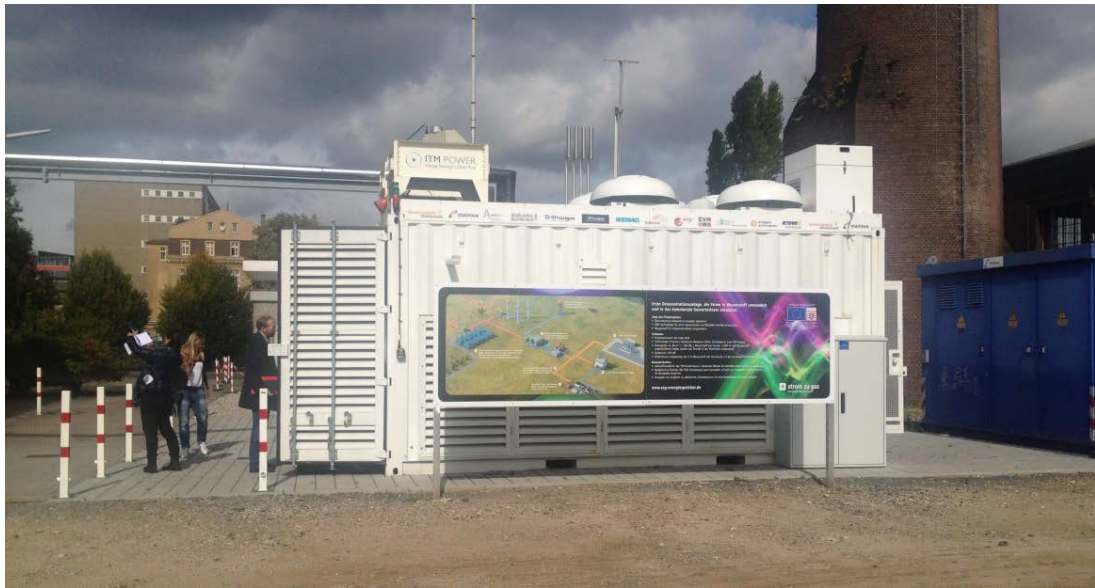
Figure 4 The picture shows the PEM-electrolyzer in Frankfurt. It is tested for a dynamic operation following a varying electricity production. The hydrogen is fed into the gas infrastructure in Frankfurt.
