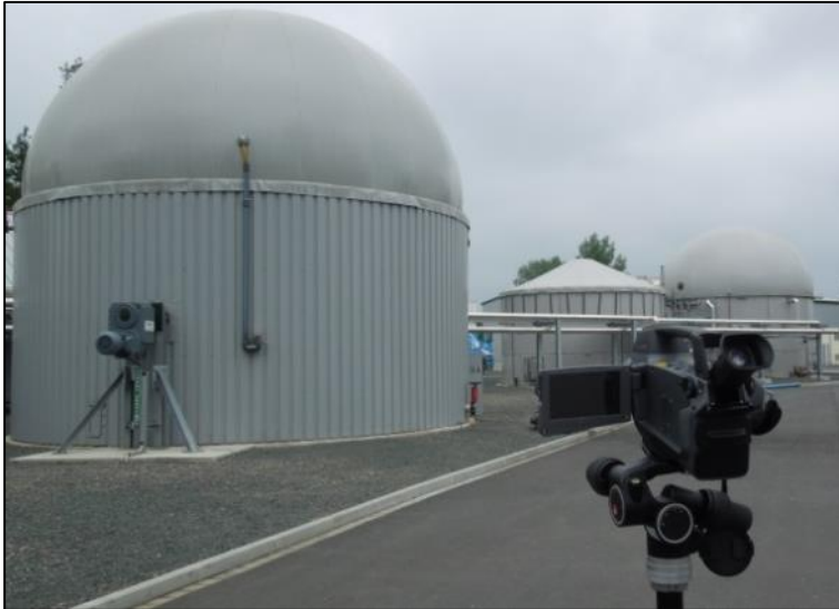
Figure 1: Infrared camera during use on the exploratory biogas plant of the DBFZ
