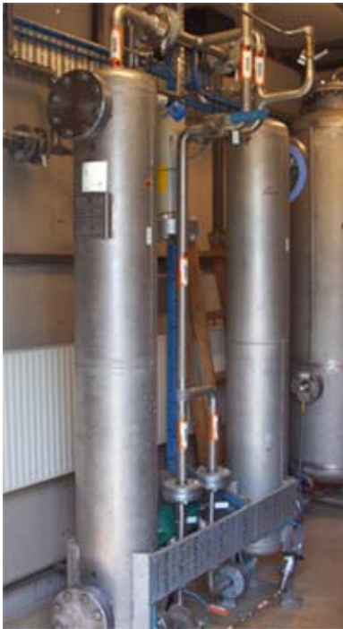
Figur 4: Adsorptionstorkar (Foto: Margareta Persson)
