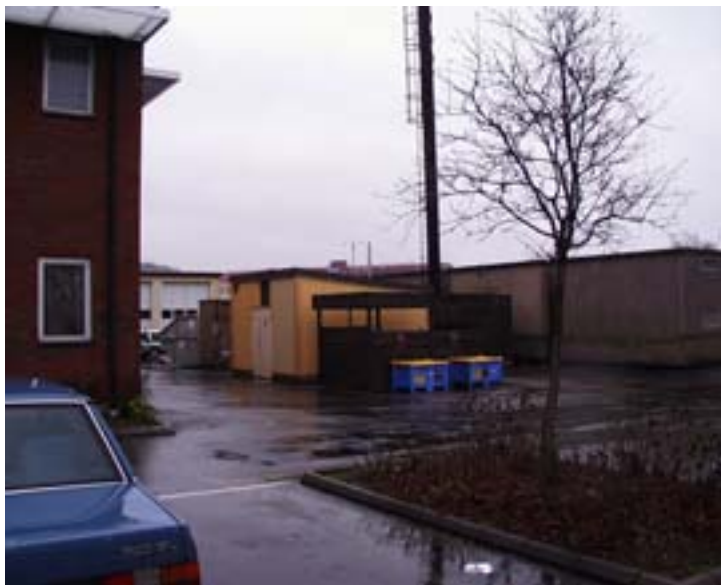
Office & warehouse with boiler house (yellow) on the right
