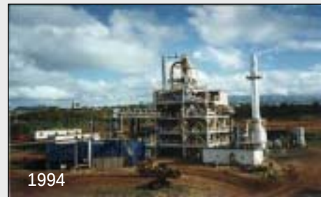
1994 100 ton per day Bioenergy Demo Plant in Maui, Hawaii using bagasse
