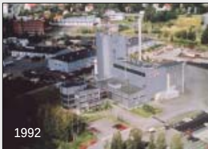
1992 80 ton per day Gasification Pilot Plant in Tampere, Finland using biomass & coal
