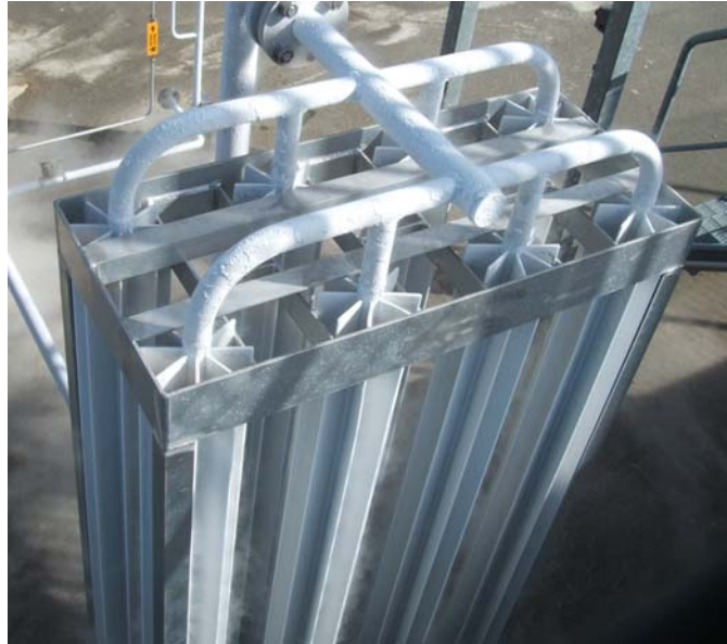
Figure 14: A fin-shaped air evaporator is used at Gasnor's LNG receiving terminal at the CCB base, near Bergen, Norway. Photo: Jens Hansson
