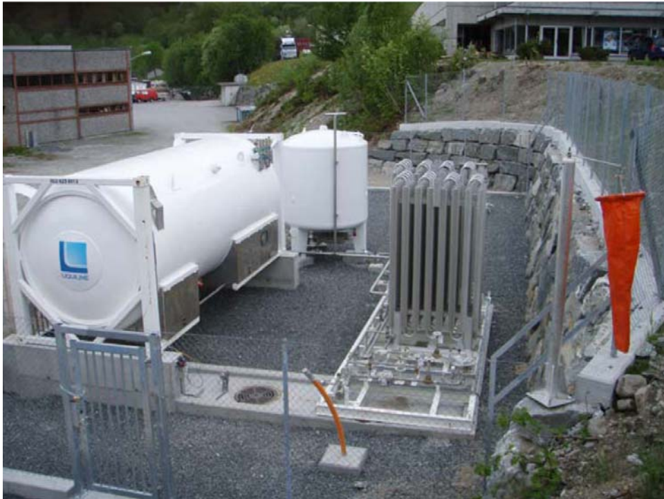
Figure 17: A Liquiline LiquiTainer® LNG storage and transport system in Norway. Photo courtesy of Liquiline AS. [44].
