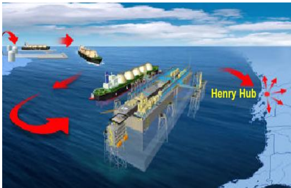
Figur 6 Proposed ChevronTexaco Port Pelican Project, offshore Louisiana - Gravity-based structure, Källa - Chevron
