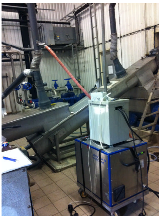
Figur 13. Photo of Deodoron connected to the ventilation air stream out from the sludge storage at Lundåkraverket.
