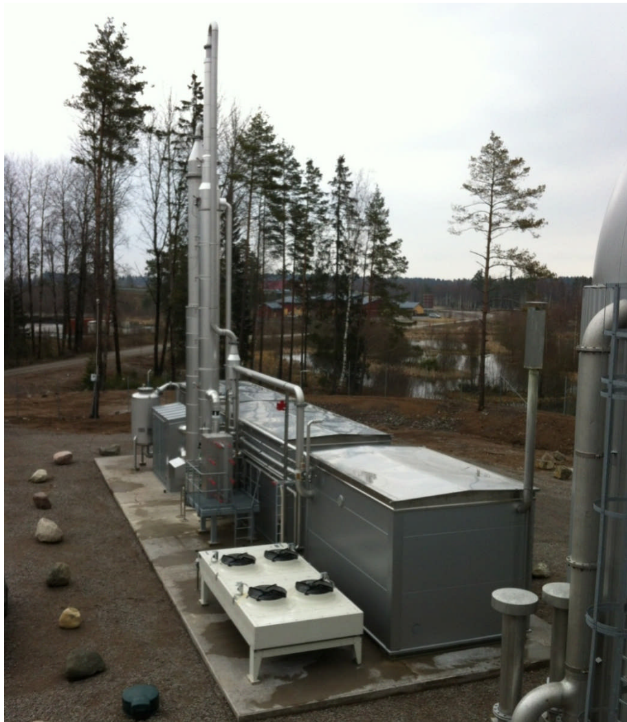
Figure 4 An amine scrubber used for biogas upgrading in Sweden. Image from Purac Puregas.
