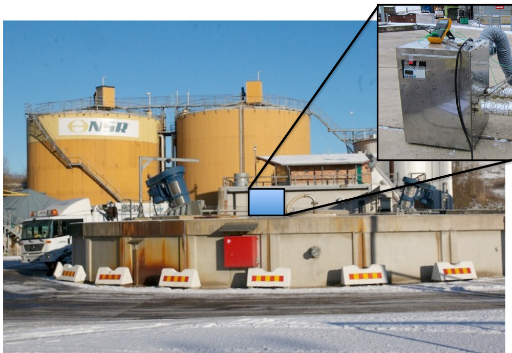
Figure 14. Installation of DEO-100 unit on top of waste material tank, at NSR biogas production plant, Helsingborg.
