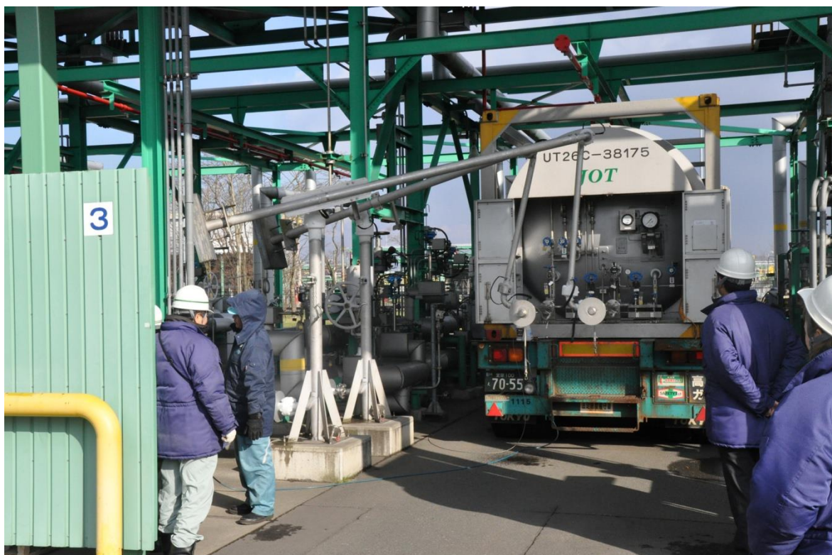
Figure 23. Loading of an LNG container at the JAPEX Yufutsu LNG plant using flexible arms. The container is located on top of a trailer. Photo: Martin Ragnar.
