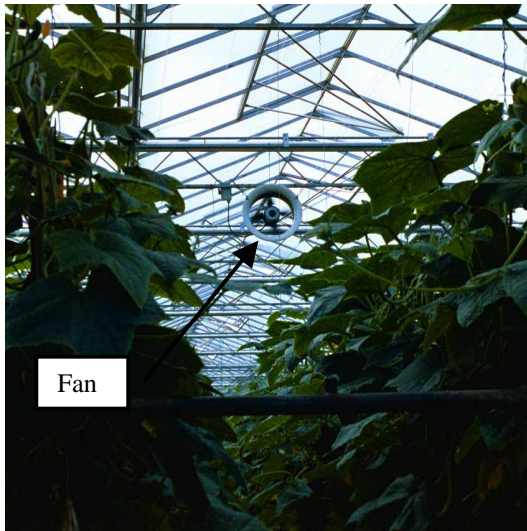
Figure 2-3. 16 fans fitted in the roof increase the air circulation inside the greenhouse.
