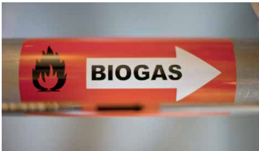
Foto: Lasse Forsberg/Biogas Systems.
